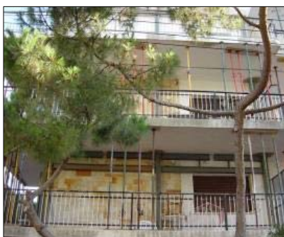
Shoring of balconies in vacation homes in Spain ( 2003)
