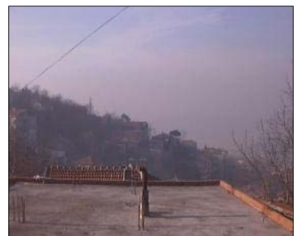
Informal living on the hills of Istanbul: Self-built houses in Beykoz (2002)
