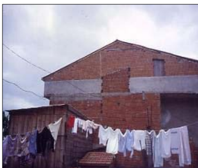
Informal living on the hills of Istanbul: Self-built houses in Pendik (2004)
