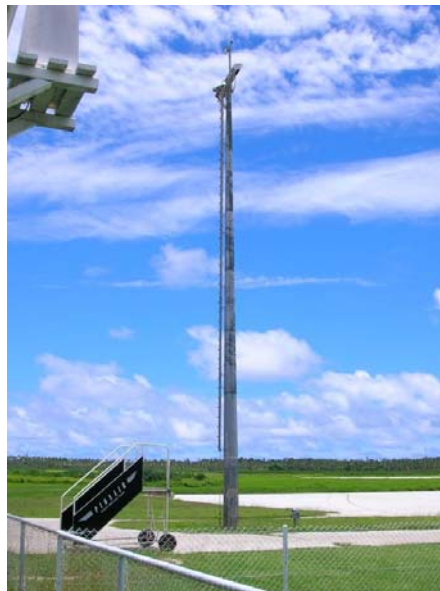
Photo 1: Lighting Standard outside Fua'amotu Met
