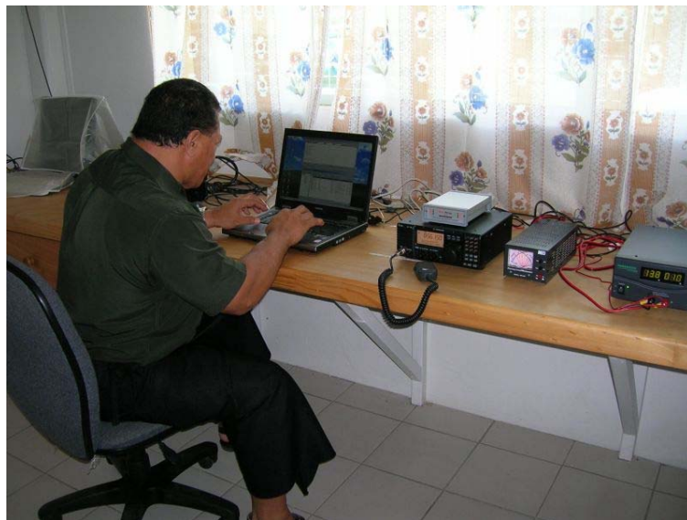
Photo 2: NEMO RANET System in Communications Room
