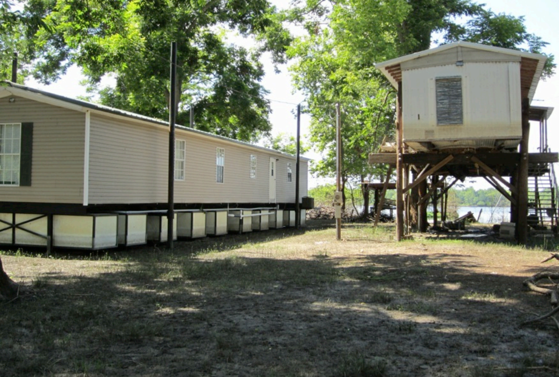
After the spring 2011 flood. Amphibious house on left is undamaged. Note waterline on elevated house on right.
