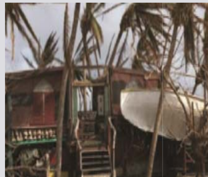
Damage after Hurricane Maria.
