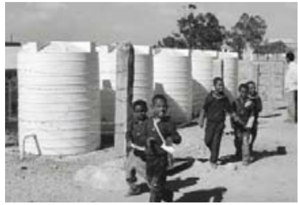
Water harvested from fog is collected in tanks. The yield can be as much as several hundred litres per day during the main fog season.
