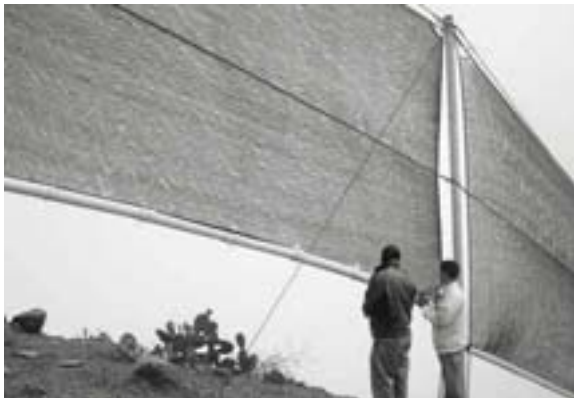
The fog nets have to withstand the strong winds that sweep across the plateau. The photo shows two workers inspecting cracks in the supports.
