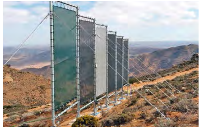
Left: The new collectors are characterised by sturdy frames and elastic rubber expanders, which are more resistant to storms. The photograph was taken during installation work in November 2013.
