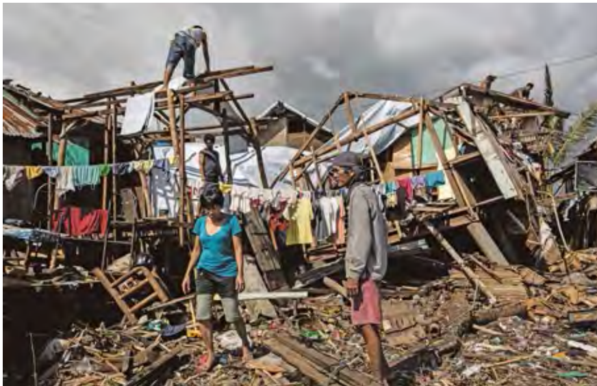
Typhoon Haiyan left a trail of destruction in its wake. Many people lost their houses. Only a few buildings in the most strongly affected areas were able to withstand the storm.
