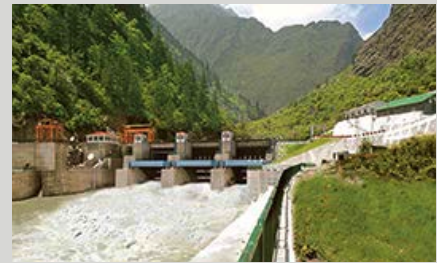
The hydropower station in Joshimath uses the natural gradient of the river for power production. This means that no dams have to be built.
