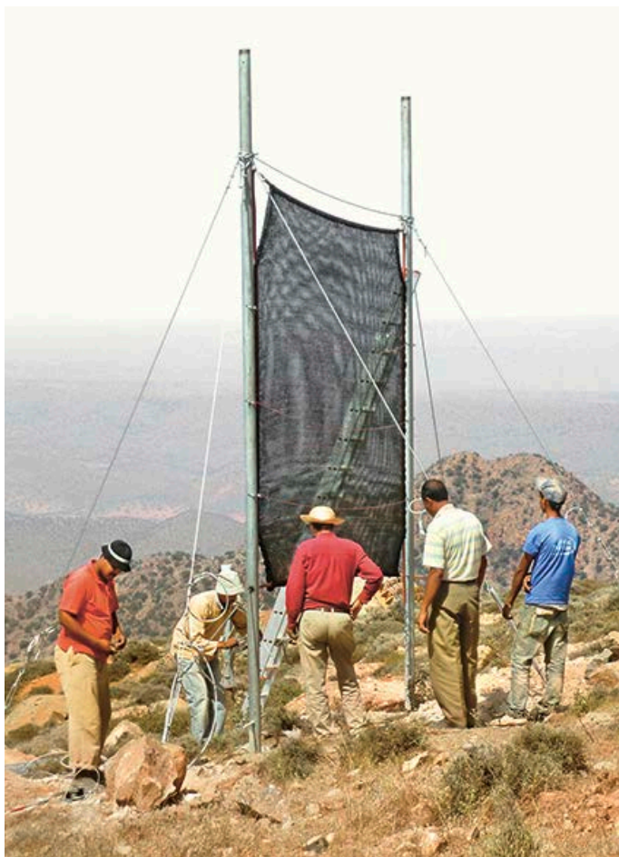
Dar Si-Hmad employees install fog collectors in Morocco's Anti-Atlas Mountains. The arid and in some parts rocky ground poses a particular challenge.
