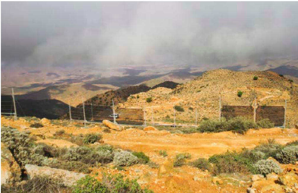
Above: Clouds of fog creep over the mountain slopes. During the foggy season, the nets can harvest more than 6,000l of drinking water from the humid air daily.
