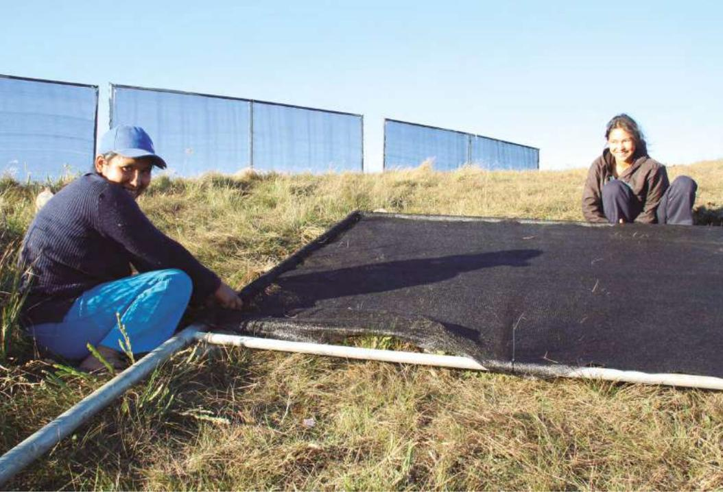
Later, in **2015**, a project was carried out with the support of the **Getxo Town Council**, consisting of the installation of fog collectors with a mesh surface area of 12 square metres. The idea was to collect large volumes of water to distribute to groups of homes located in remote areas that have difficulty obtaining water by other means.
