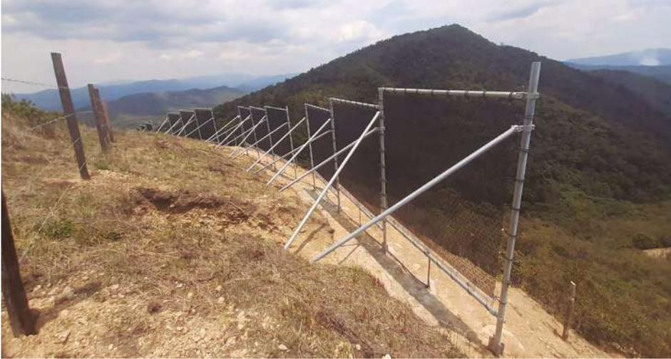
Figure 11. Diagram of the fog collector system at the Sivingalito site
