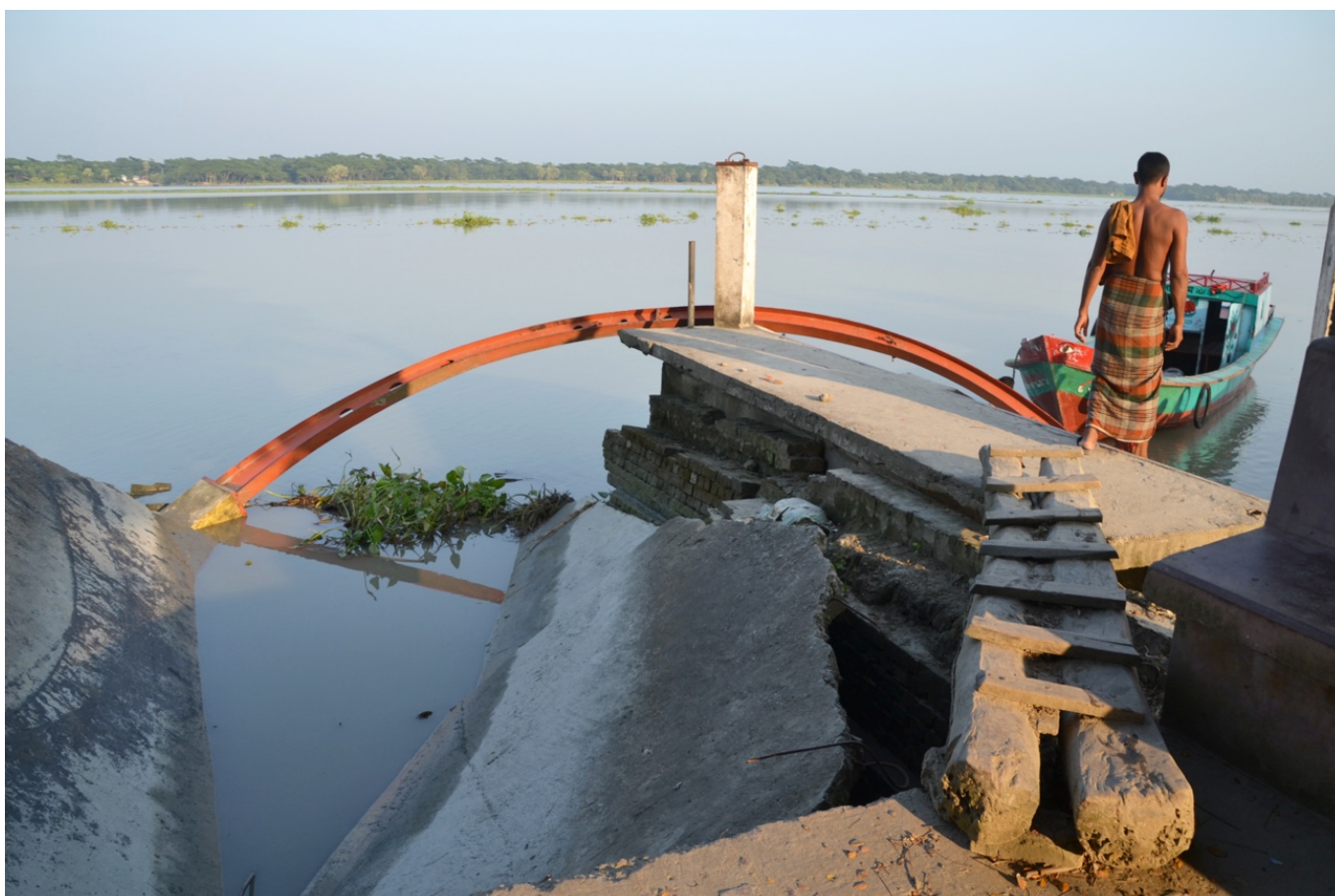
The only harbour on Mazer Char finally collapsed due to the riverbank erosion (© Sonja Ayeb-Karlsson).
