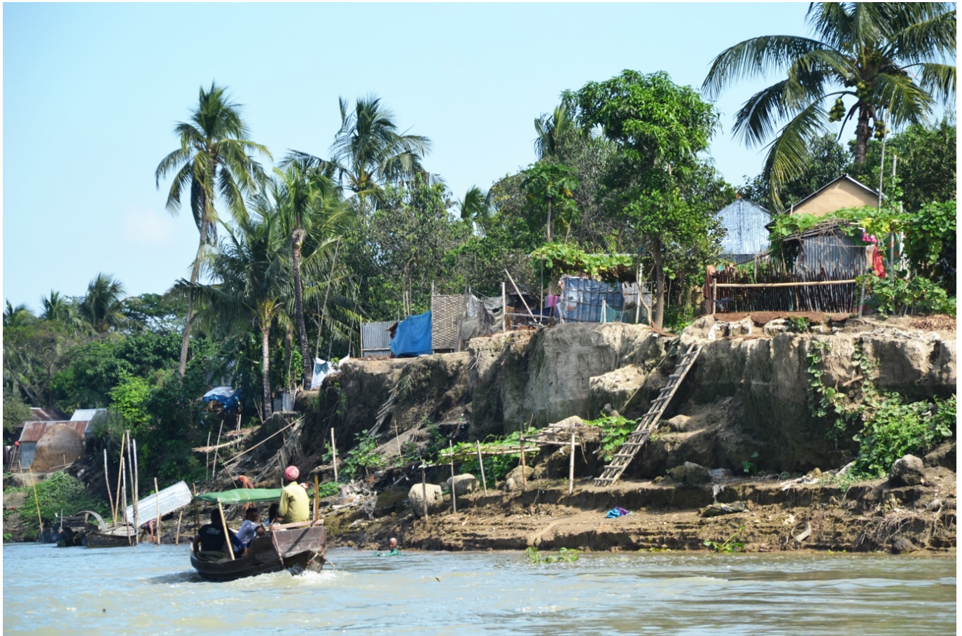
People end up losing home after home to the riverbank erosion in Singpur (© Sonja Ayeb-Karlsson).
