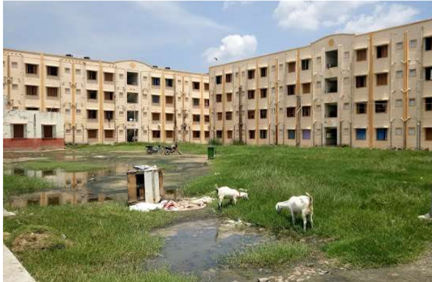
Post-tsunami resettlement colony in Chennai, built on wetlands and prone to flooding. Photo by C Singh
